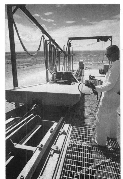
CONTROLLING progress of test cart as it moves up incline is Gerry Gay (7325-2). Results of test will be traced by recording oscillographs in instrumentation building nearby. Facility has been operating since June.
